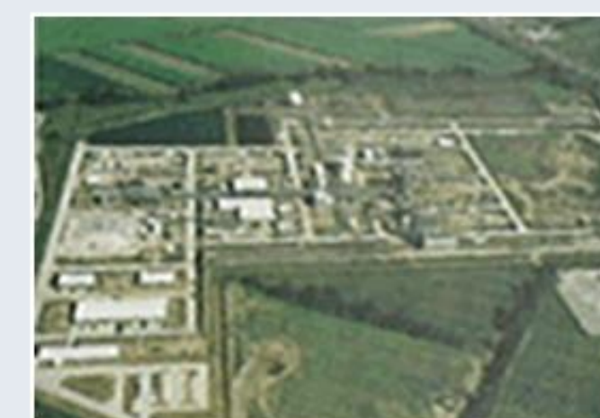
Addis Plant, Shintech Inc.
